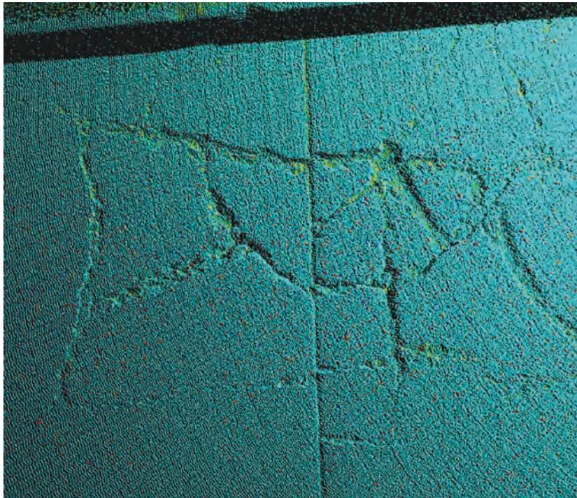
**Figure A-16: Intensity return used to highlight concrete cracking in a static scan (plan view).**
